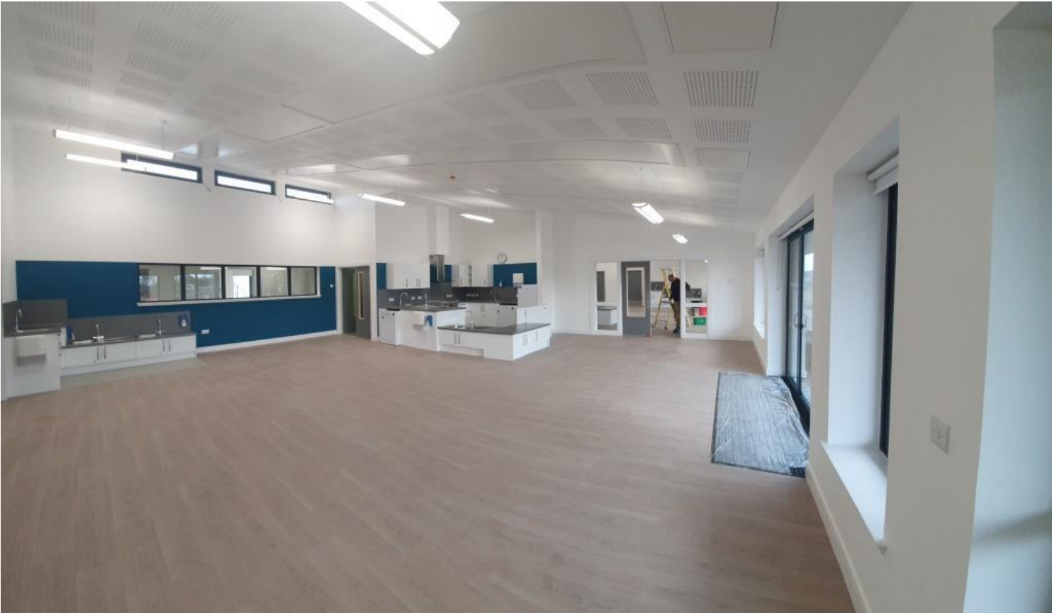
Kingsford Nursery – Nearing Completion – Internal
