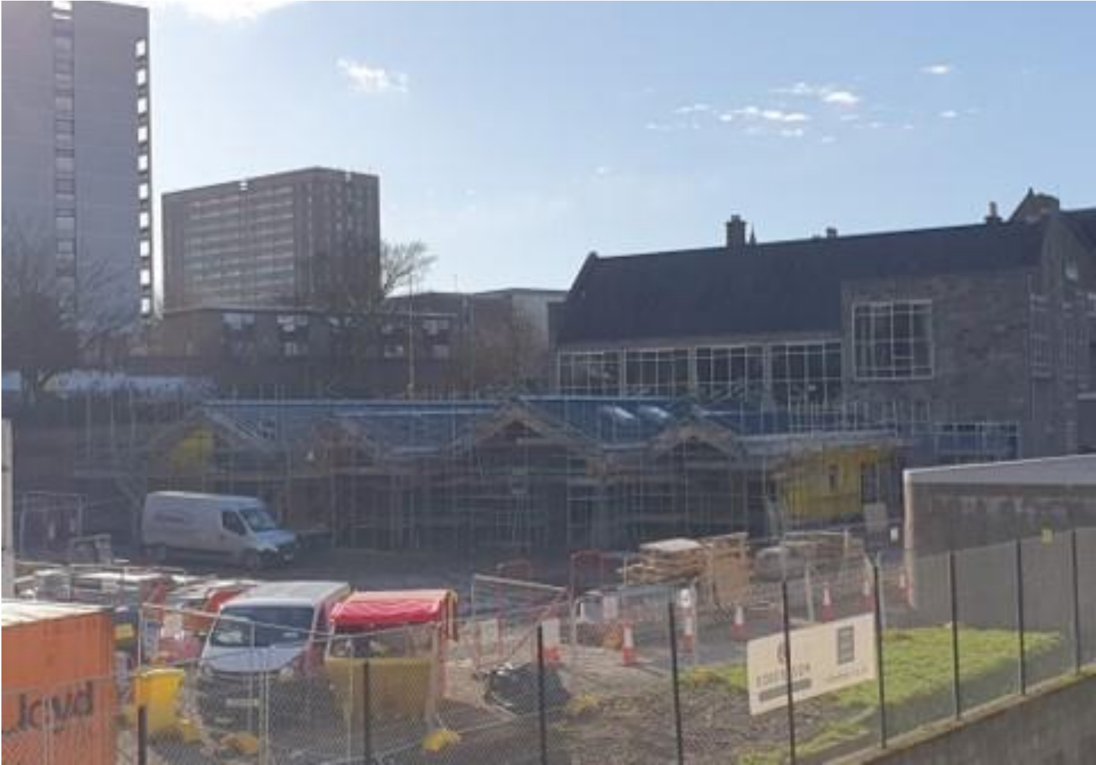
Gilcomstoun Nursery – General Progress
