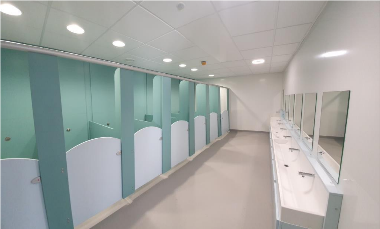
Tillydrone Nursery – Nearing Completion – Internal
